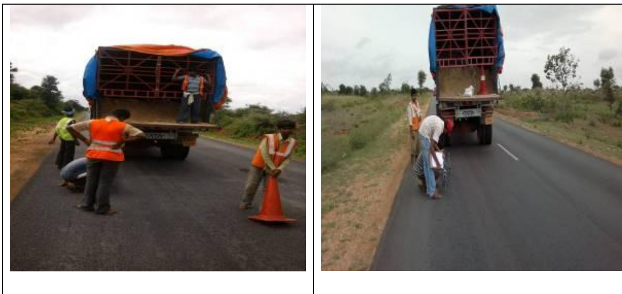
Figure 6-1: Photographs showing BBD Tests in Progress
