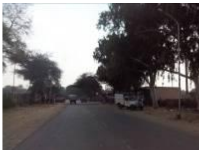
Good Condition @ km 6.5
